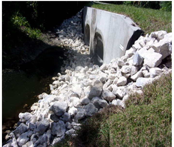
Neighborhood Drainage Improvements
