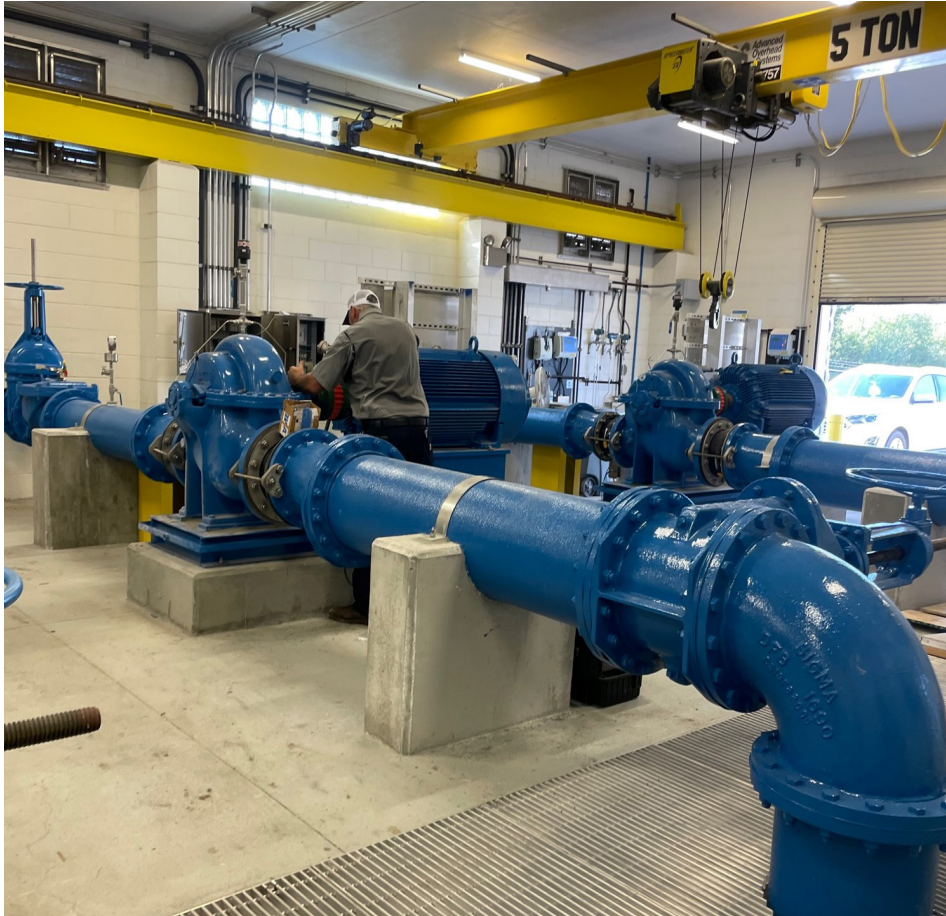
A County employee works on pipes in the South County Pump Station.
