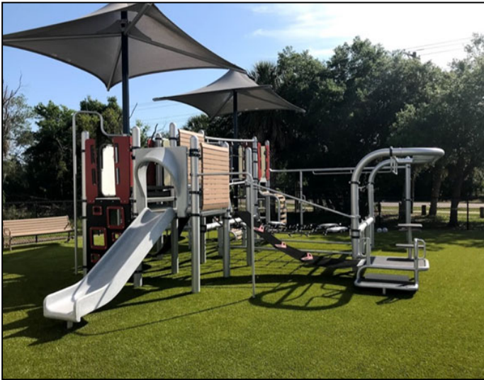
Park Playground Replacement
