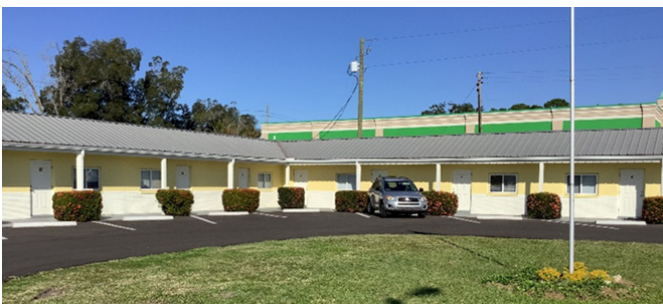
The former Carol Motel was transformed into Las Villas, a multifamily rental property for people emerging from homelessness.
