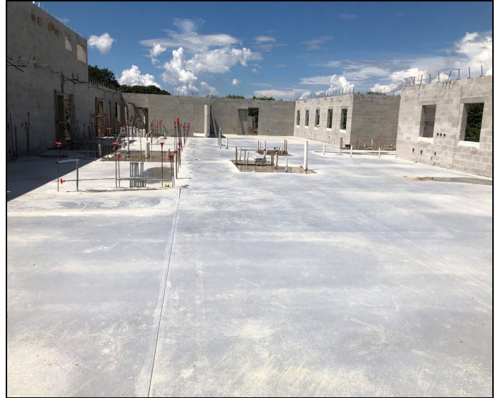
Apollo Beach Fire Station #29 Under Construction
