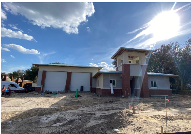
The new Central Brandon Station nears completion.
