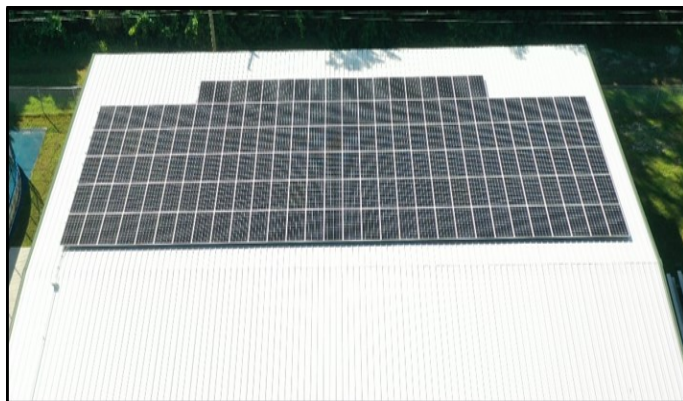
Solar Panels – Ruskin Recreation Center
