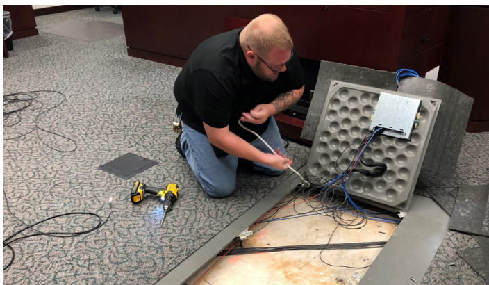
Court IT staff reconfigure wiring to create social distancing in the courts.
