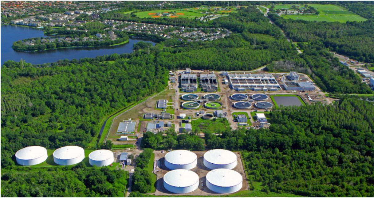
The Northwest Reclaimed Water Facility is shown.
